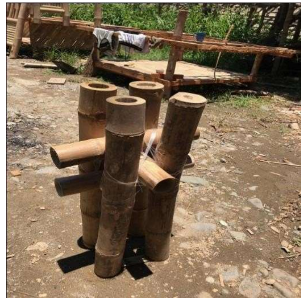
Fig. 4. Column and Beam Connection.
