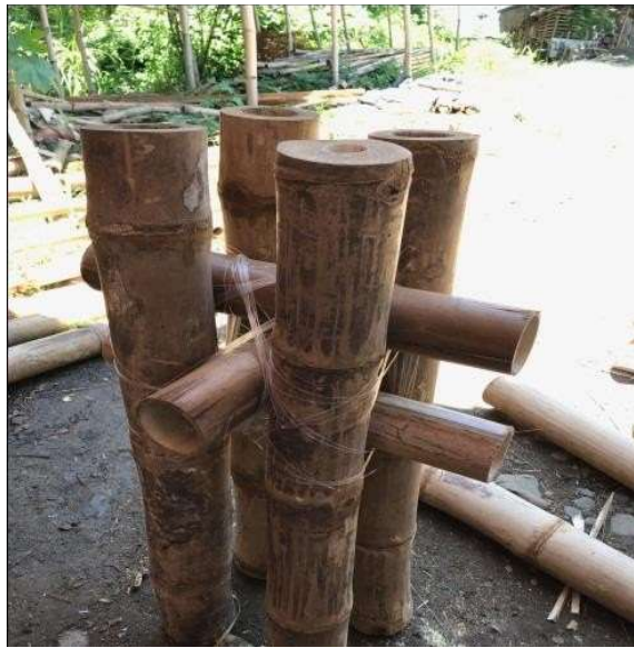
Fig. 5. Column and Roof Connection.
