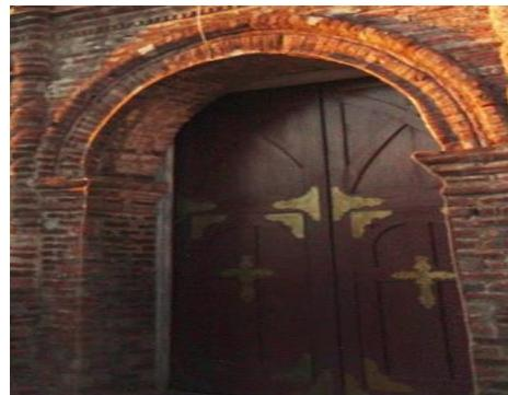
The rest of façade features the restored bricks and symbols engraved on it. The bricks are purely stretched which laid horizontally with its length in the direction of the free of the wall. It was formed as stretcher bond wherein all causes laid as stretcher with the vertical joints of one course falling midway between those of adjustment causes. At the edge of the façade, a classical European pattern has also formed.
